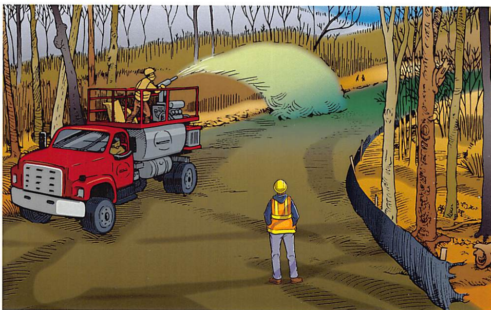
Figure 5. Hydroseeding.
